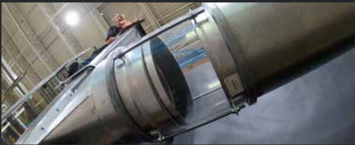
WITH AN INTEGRATED SPARK TRAP
